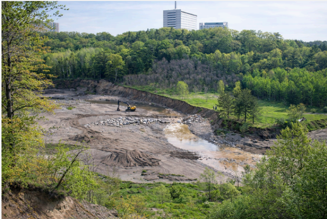
Highland Creek sewer protection in Toronto, Ontario
